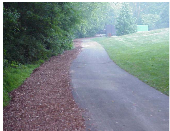
Figure 1.18: Temporary access road widening
