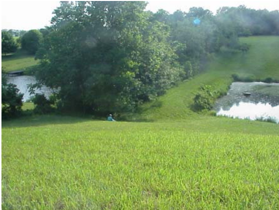
Figure 1.11: Woody vegetation on embankment
