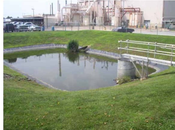
Figure 1.6: Riser without trash rack
