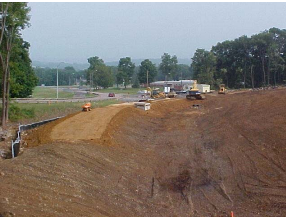
Figure 3.4 Dam construction – Photo 3
