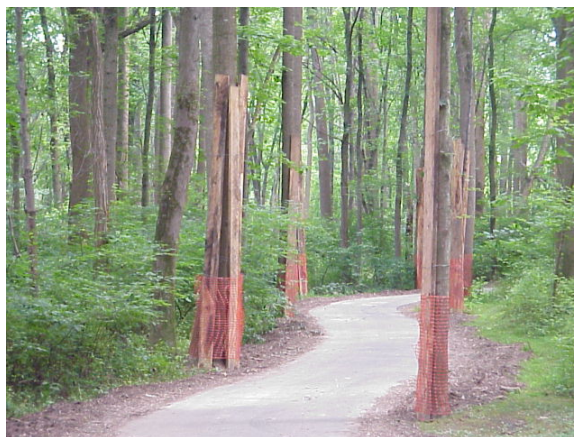
Figure 5.23: Tree scar protection
