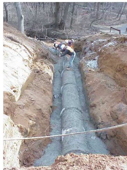
Figure 3.1: Barrel laid in concrete cradle
