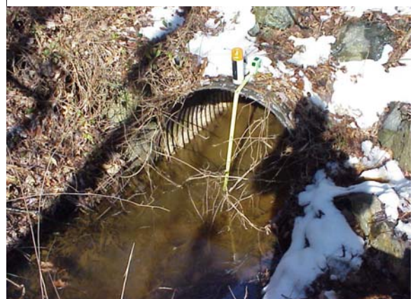
Figure 5.22: Forced access location.
