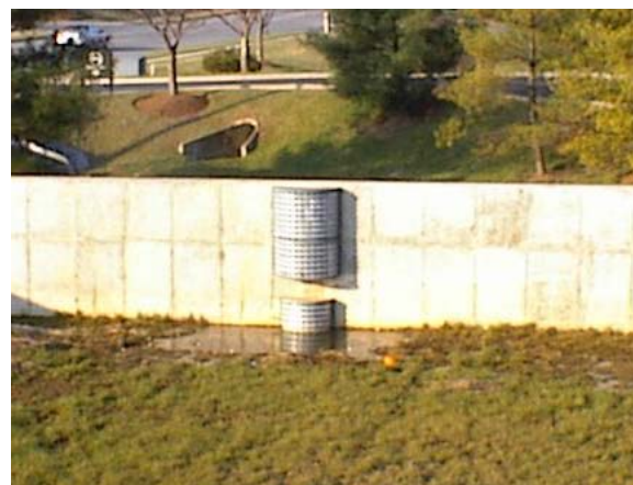
Figure 2.2: Half round CMP low flow opening and trash rack
