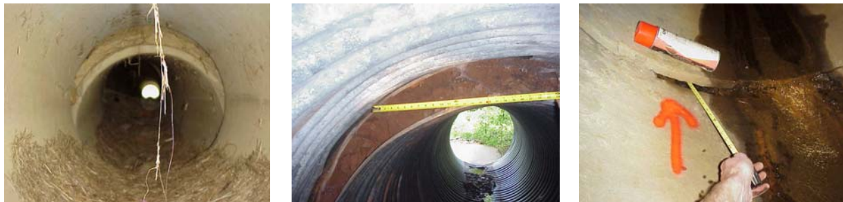
Figure 5.7: Misalignment in RCP (left and right) and CSP (center) applications.
