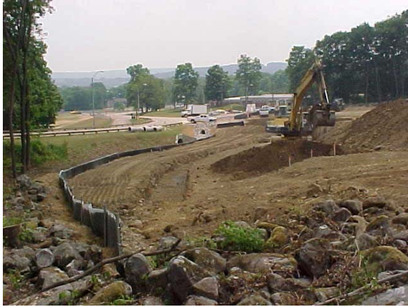
Figure 3.2: Dam construction - Photo 1
