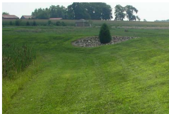
Figure 5.14: Unwanted vegetation - tree on embankment
