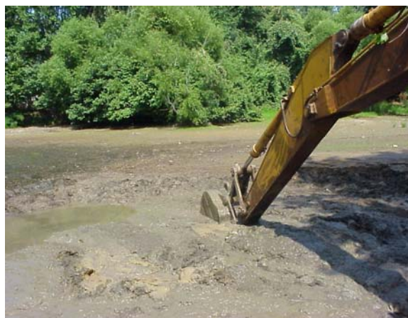
Figure 5.19: Mechanical dredging with backhoe.
