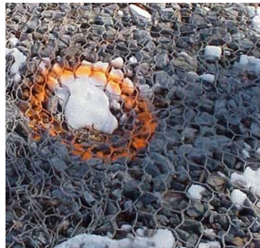
Figure 4.4: Marking a hole in gabion fabric
