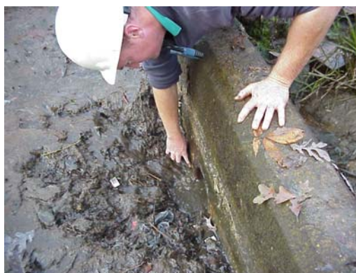
Figure 5.4: After clog is removed
