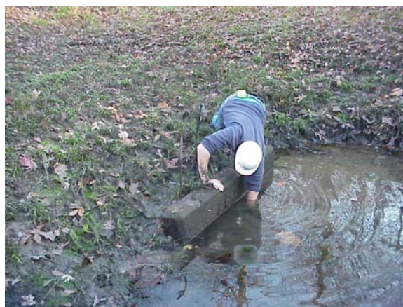
Figure 5.3: Clogged low flow orifice (before maintenance)
