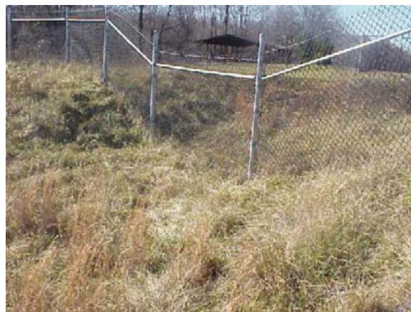
Figure 2.1: Fence across Emergency Spillway
