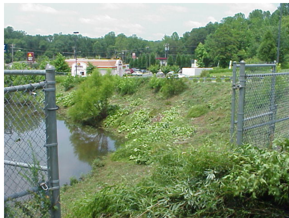
Figure 2.6: Chain link fence
