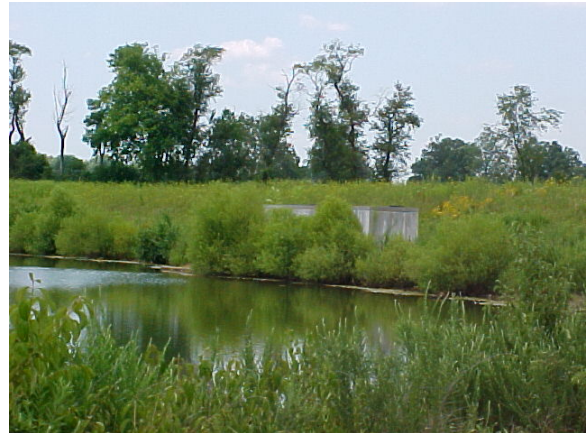
Figure 1.12: Excessive vegetative growth obscures riser
