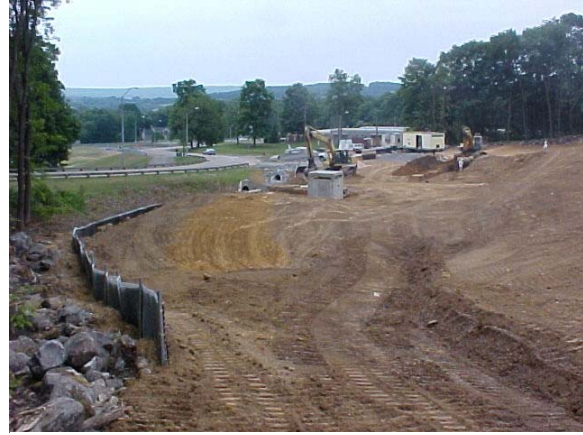
Figure 3.3 Dam construction – Photo 2
