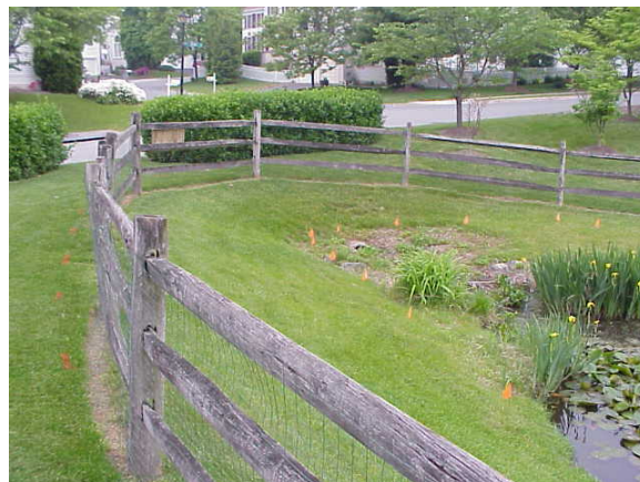
Figure 2.7: Post and rail with mesh backing
