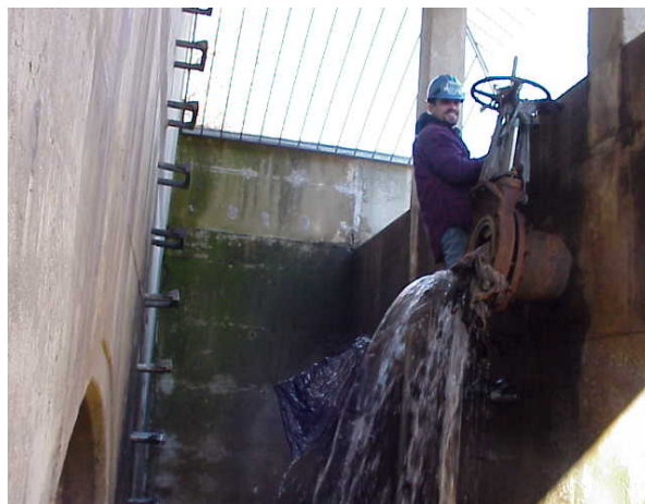
Figure 5.2: Clogged valve
