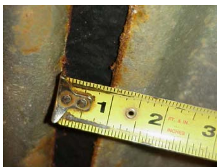
Figure 5.5: Improper pipe joint but rubber seal is visible.
