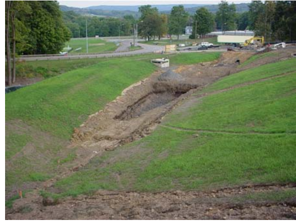
Figure 3.5 Dam construction – Photo 4
